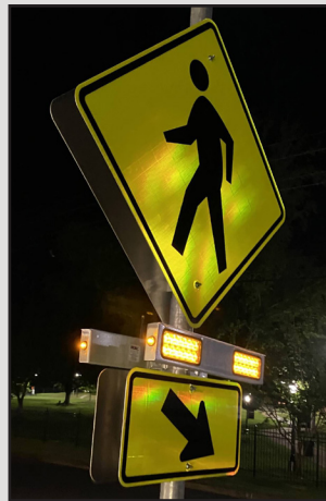
Example photo of a rectangular rapid flashing beacon to improve pedestrian safety.
