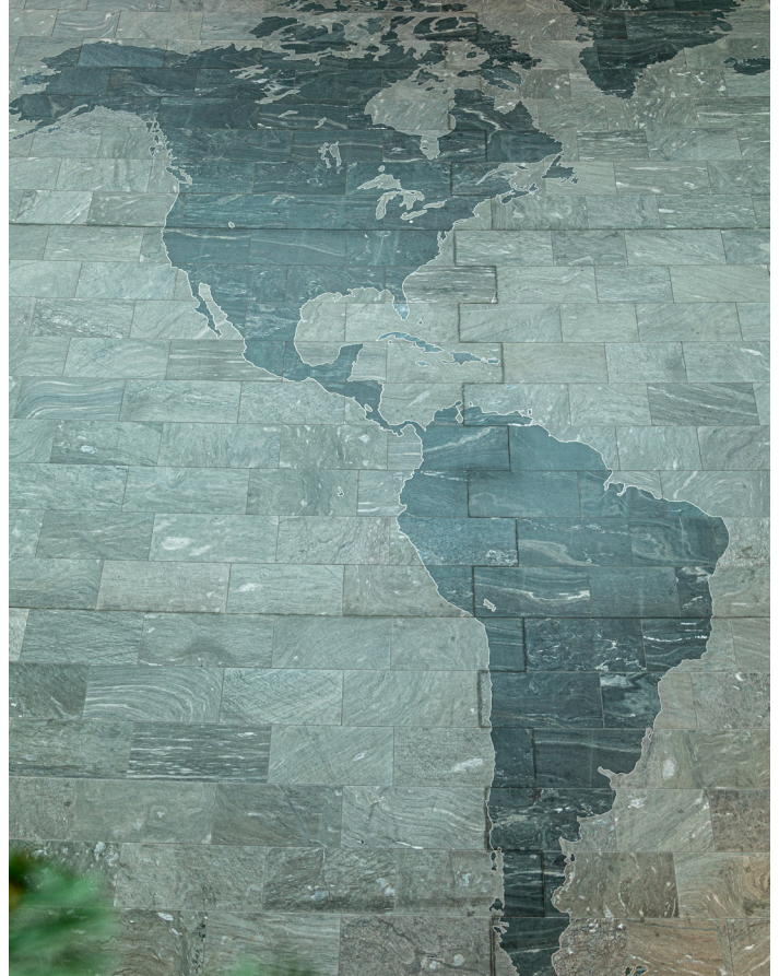
Flooring, created with Vals Quartzite, quarried and fabricated into rectangular pieces in Switzerland. The stone was shipped to Creative Edge in Fairfield, Iowa, where it was cut into the world map pieces and stainless steel edging was installed outlining the continents. The fabricated pieces were shipped to the Beachwood project site and installed by Corcoran Tile.
